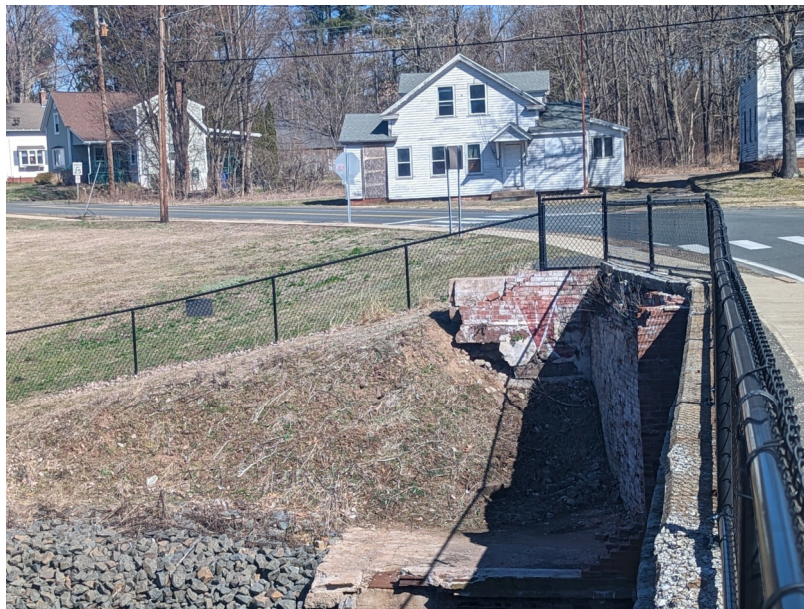
Old Building Wall Remnants & Fence Barrier
