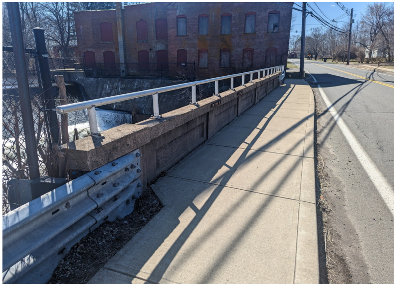
Sidewalk & East Parapet
