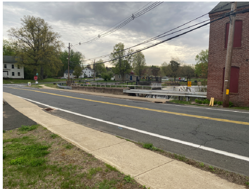
Bridge Travel Way
